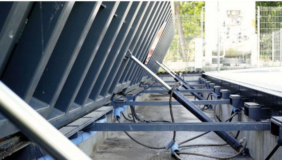
THE BARRIER IS MOUNTED IN THE RECESS.
