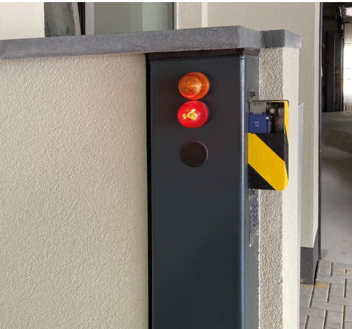
EMERGENCY LIGHTING AND END SWITCH FOR BARRIER CLOSURE.
