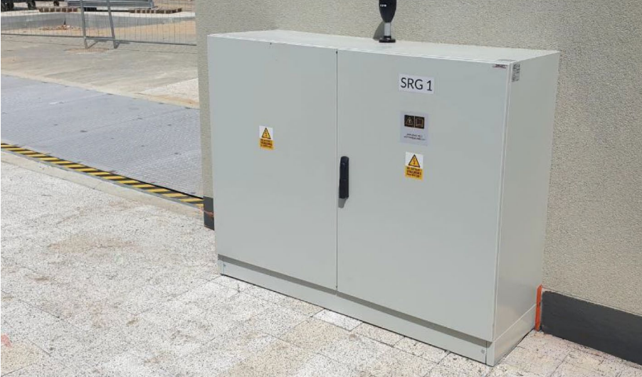
STEEL CABINET WITH POWER AND CONTROL SYSTEMS.
