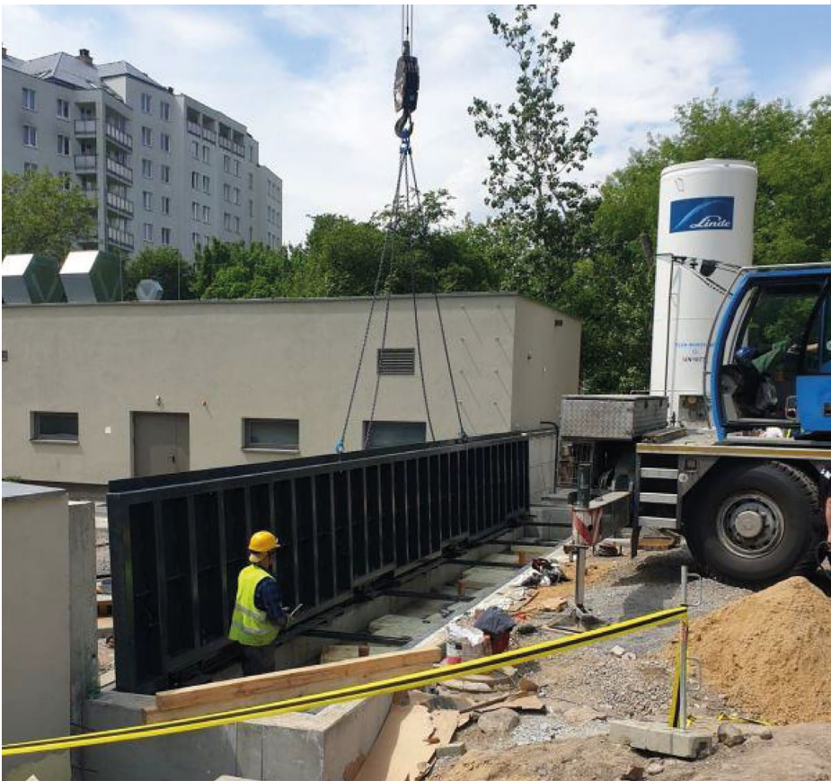
THE MOBILE PLATFORM IS INSTALLED.
