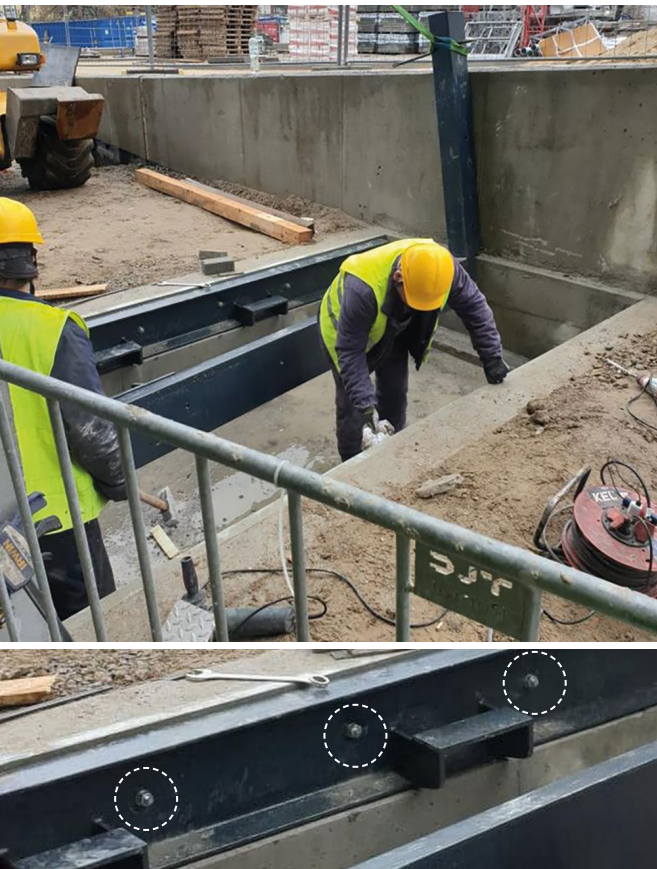
THE STEEL STRUCTURE IS MOUNTED USING EXPANSION ANCHORS.
